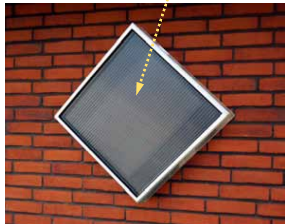
The SV2 can be mounted like this - we call it the "Diamond model"
