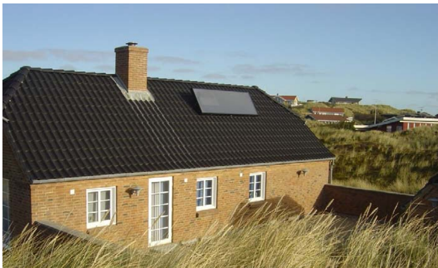
On this picture you see a 3m 2 system (SV30) on the roof. The collector is placed on stands in an angle of 60°. This angel gives the optimal effect the whole year round.
